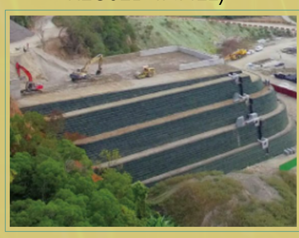
ABUTMENT (GEOSYNTHETIC REINFORCED SOIL WITH REUSED INFILL)
